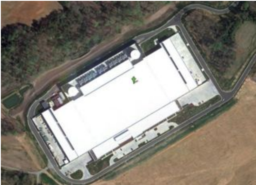
Apple's 1 billion dollar datacenter in North Carolina
