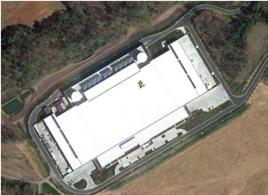
Apple's 1 billion dollar datacenter in North Carolina
